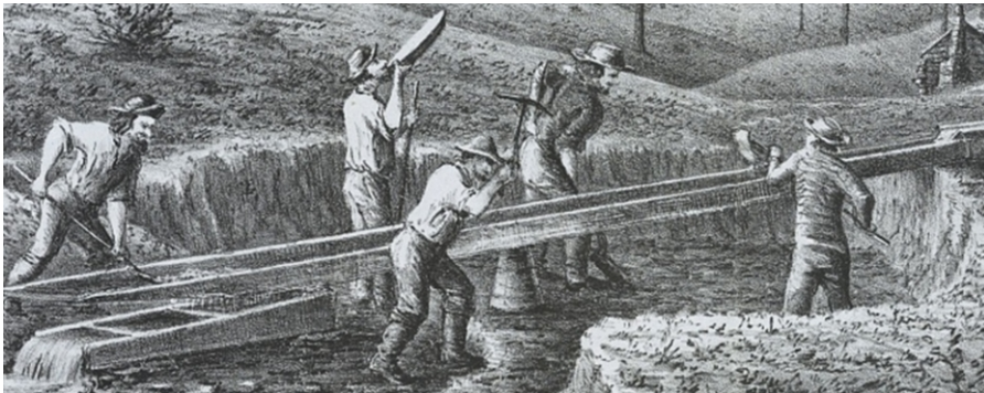
miners working the sluice (long tom) as described in letter
