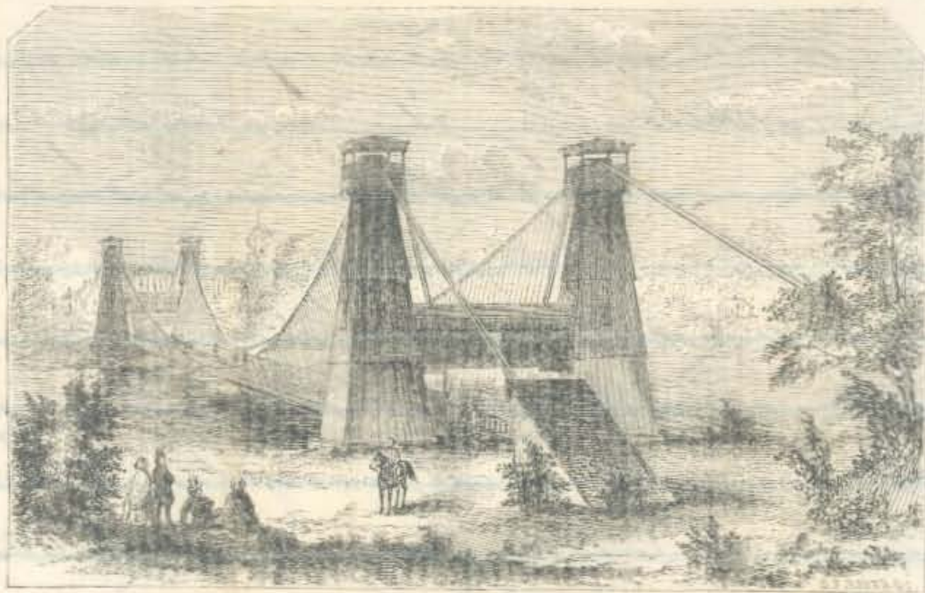
SUSPENSION BRIDGE BETWEEN ST. ANTHONY, MINNEAPOLIS, MISSISSIPPI RIVER.
