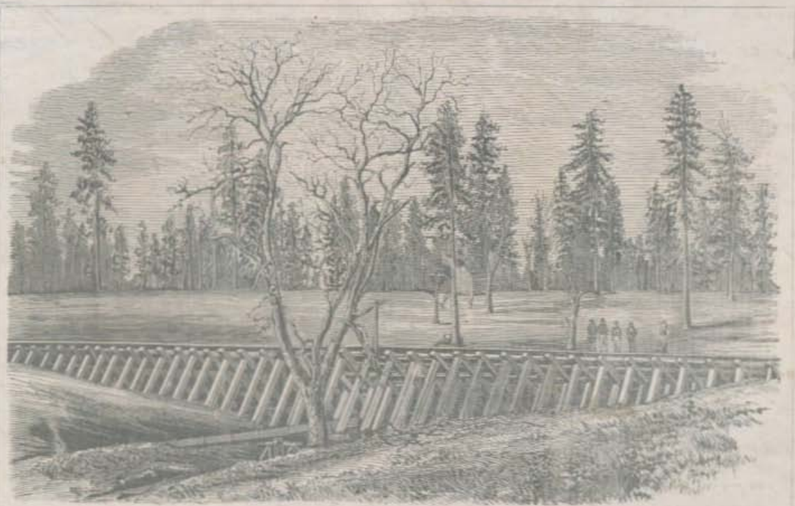
PILOT CREEK CANAL, GEORGETOWN, EL DORADO COUNTY.
