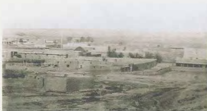
General View of Fort Craig Looking South, Circa 1870's
